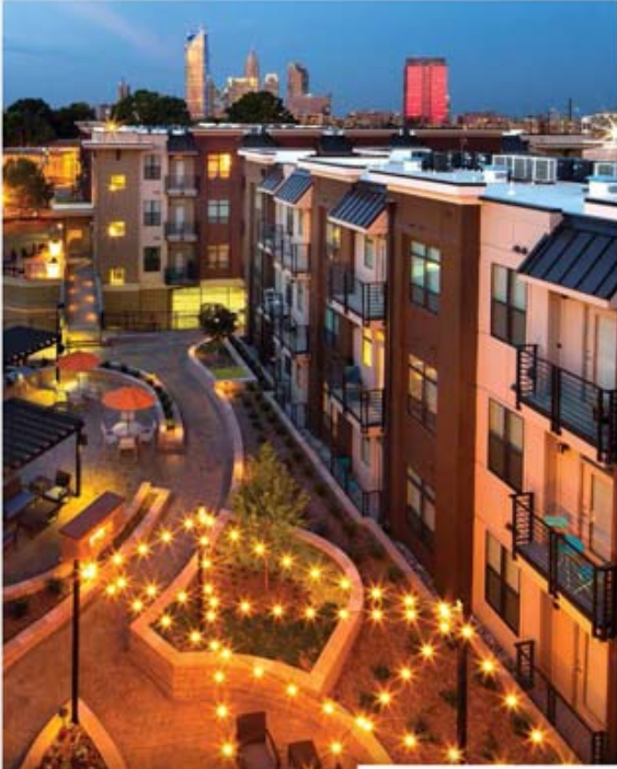
Park & Kingston Apartments | Charlotte, NC
